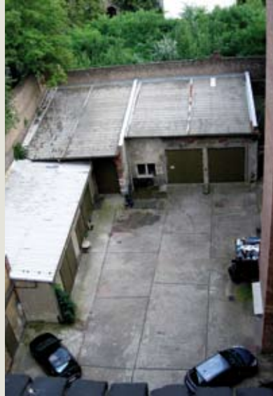
Hinterhof Back courtyard
